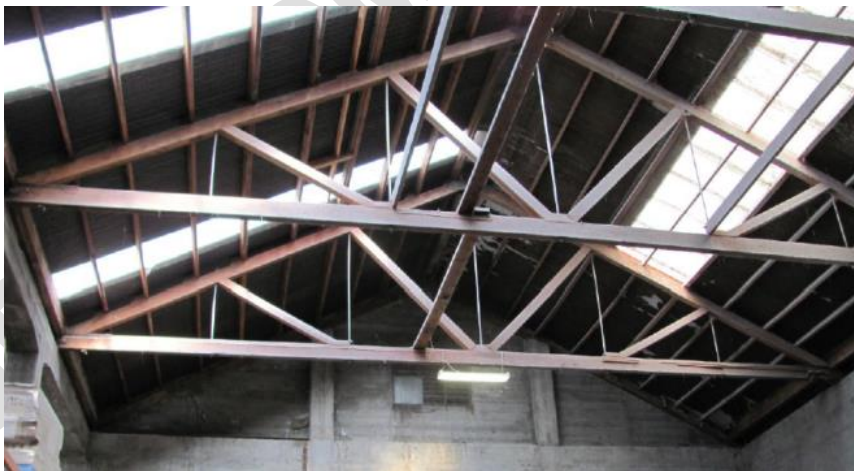
Figure C2E.1: Example of a flexible diaphragm
