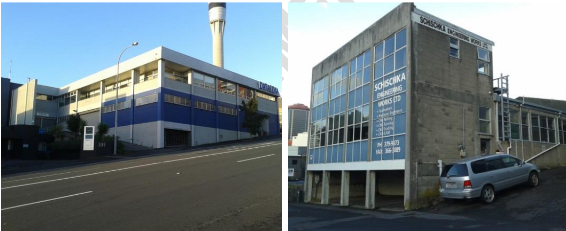
Figure C7.4: Examples of reinforced concrete frames with concrete block masonry infill (Laura Putri)
