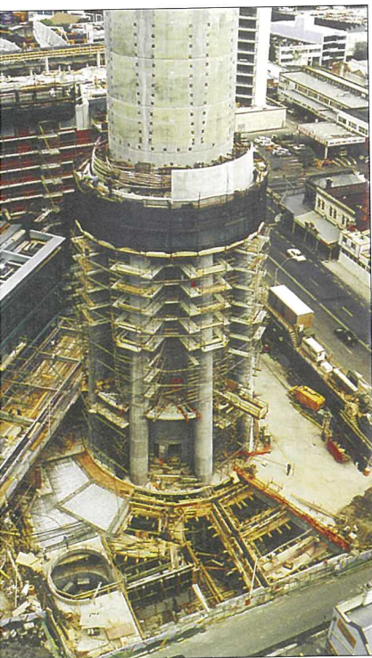
Above: Ducts and anchorage boxes from outside the shaft.
